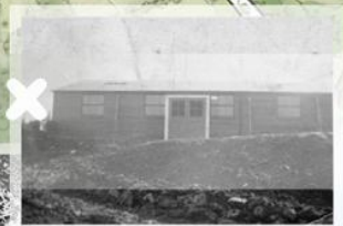
The WI Hut under construction, 1925
